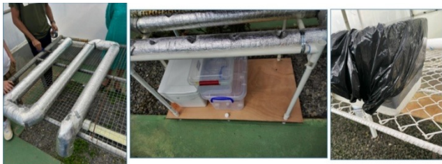
Figure 8. PVC pipe cover (left and middle) and tank wrapping (right).
